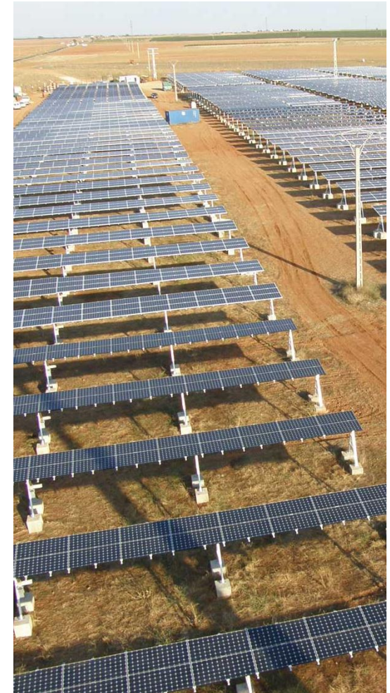
European Energy Solar Park Villaneuva, Spain
